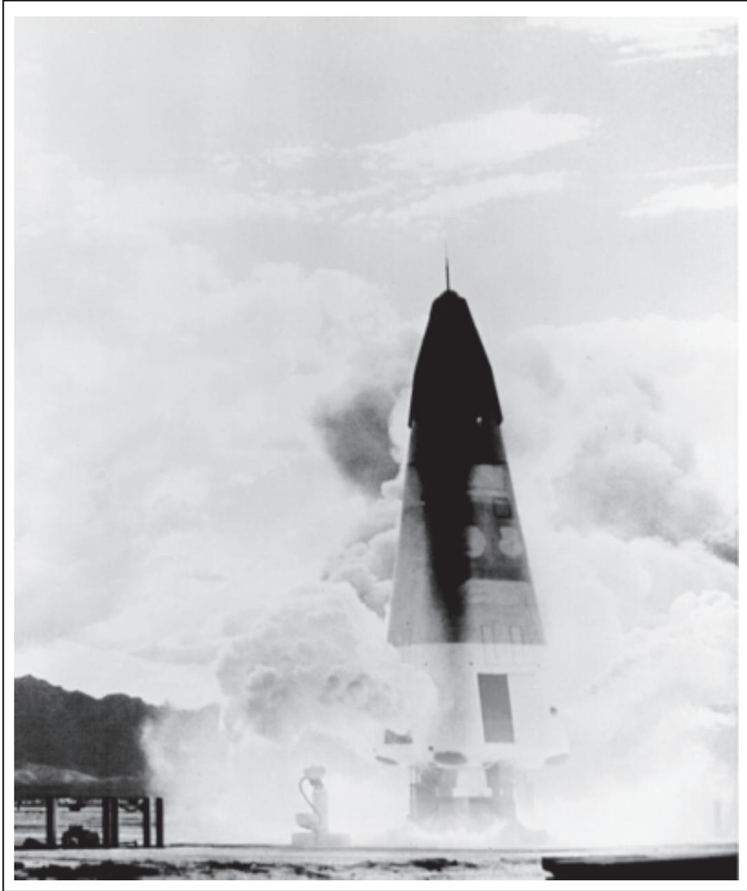
The Delta Clipper Experimental (DC-X) vehicle, originally developed for the Department of Defense, lifts off at the White Sands Missile Range in New Mexico. NASA has assumed the role of managing the vehicle's further development. The DC-X lifts off and lands vertically. NASA hopes this vehicle could lead to a low-cost payload launching system. The Delta Clipper was recently renamed the "Clipper Graham" in honor of the late space pioneer Lt. General Daniel O. Graham.
